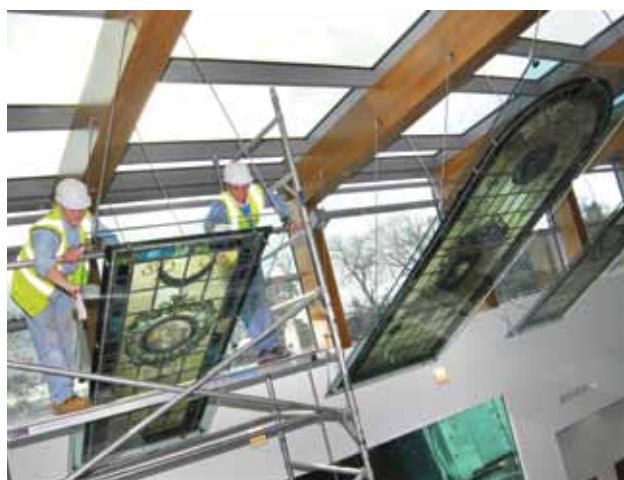
The Summerhall windows being carefully installed in the new atrium.
