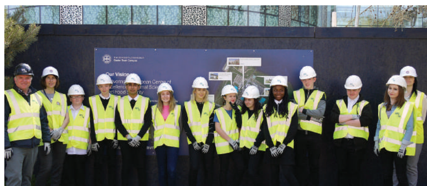
The pupils were given the chance to visit the Campus Hub which is currently under construction.
