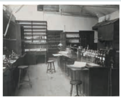
Teaching laboratory at Clyde Street. The premises underwent extensive refurbishment in 1833 to provide purpose-designed facilities.
